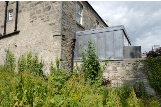
Image 05 – Rear corner of gable with garden wall and existing rear extension
